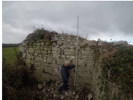
Fig 09: Recent loss of stone on west elevation and ivy roots on wall tops visible
