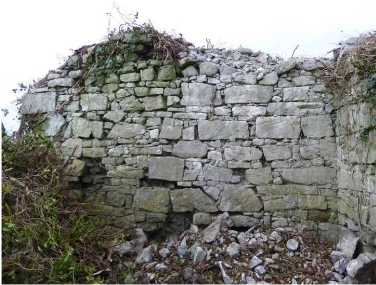
West elevation, internal face – Recent collapse evident on the wall top. Pockets of facing stone lost at low level
