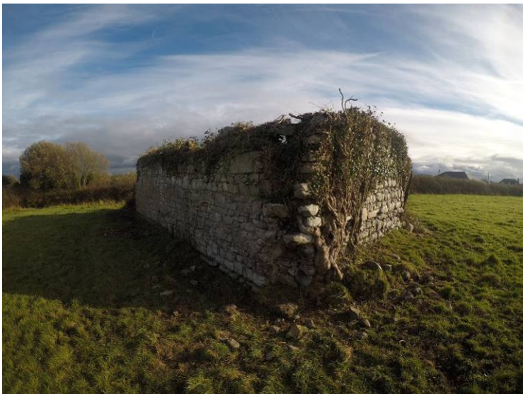
North west corner – Loss of corner stone clearly visible. Ivy roots visible along wall top of both walls
