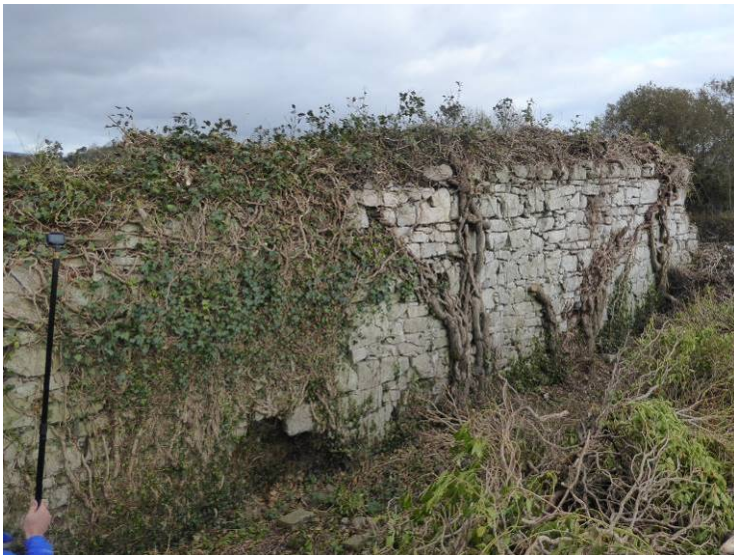
North elevation, internal face – Pockets of stone lost and extensive ivy coverage in areas.
