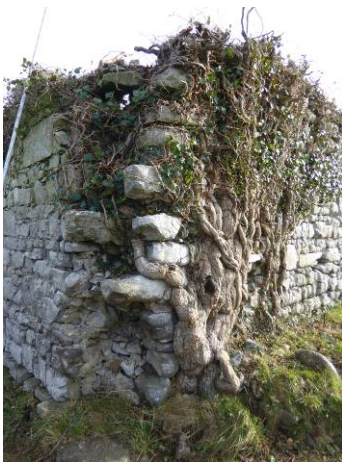
Fig 08: Connection between north and west elevation compromised
