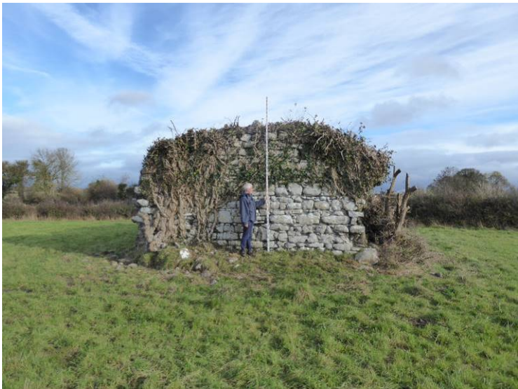
West elevation – stone lost at each corner and along wall top. No evidence of original building height
