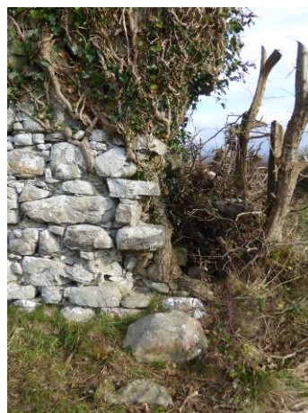
Fig 07: Trees growing from base of wall, high level stone not supported
